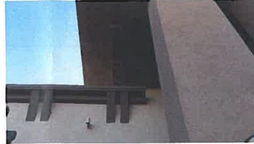
2 SAFEWAY STORE - MAIN ENTRY CORNICE
