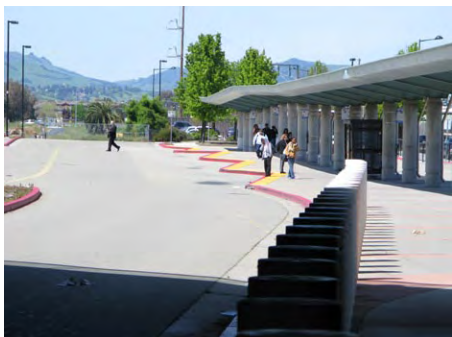
View from underneath I-580 overpass looking north Figure 33
