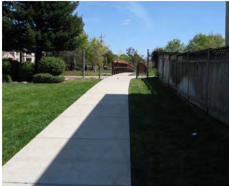
Existing bridge to be utilized to cross Tassajara Creek Figure 21
