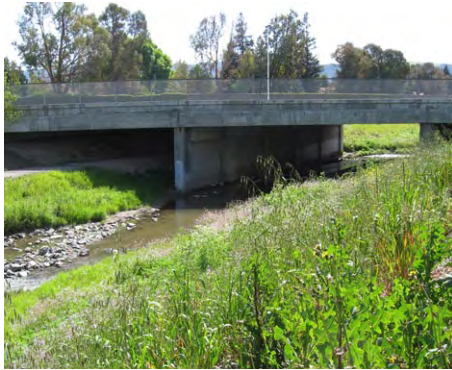
Existing bridge at the proposed Arroyo Mocho trail crossing Figure 20
