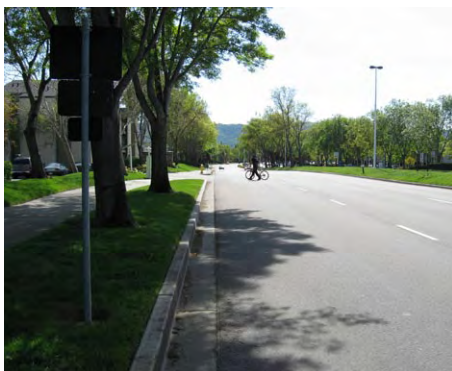
Existing conditions at West Las Positas Blvd.
