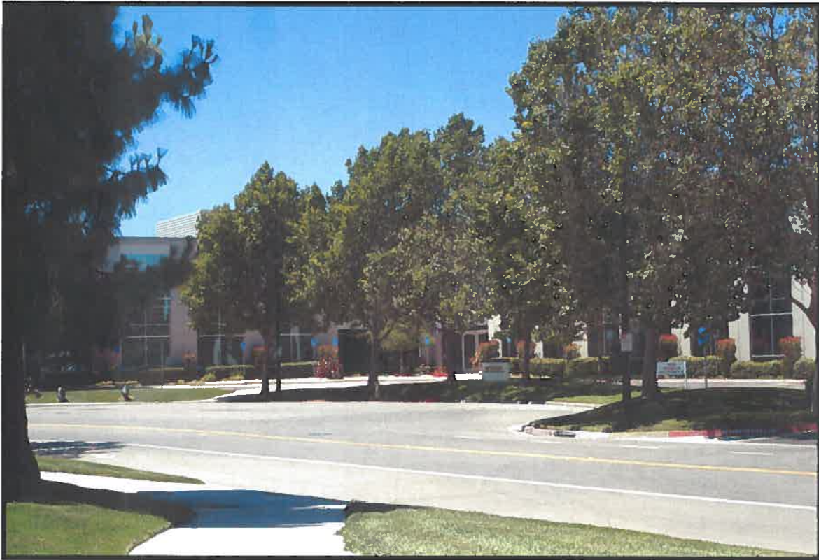
Figure 7, 6100 Franklin Drive, Northwesterly of the Project Site.
