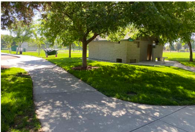
Existing, non-ADA compliant restroom.
