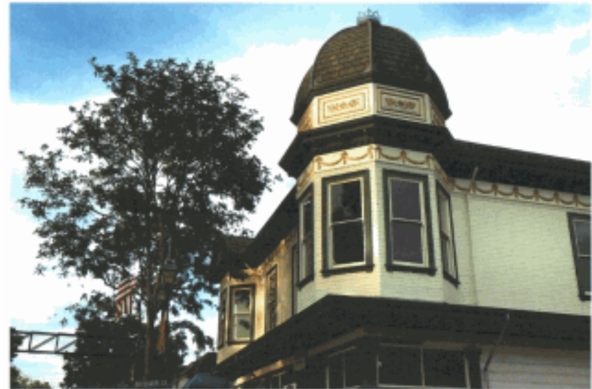
Former Kolln Hardware store during renovation
