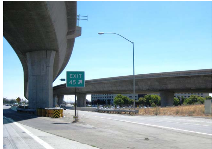
Flyover connections from I-680 to I-580
