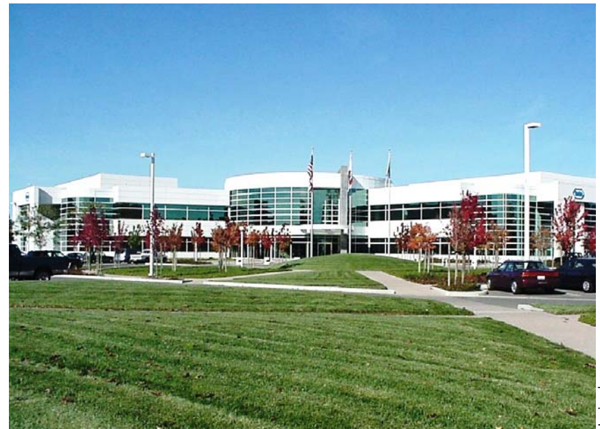
Roche Molecular Systems building in Hacienda Business Park
