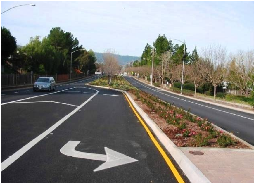
Vineyard Avenue roadway improvements
