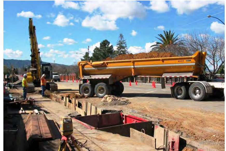
Maintenance of utilities in street right of way
