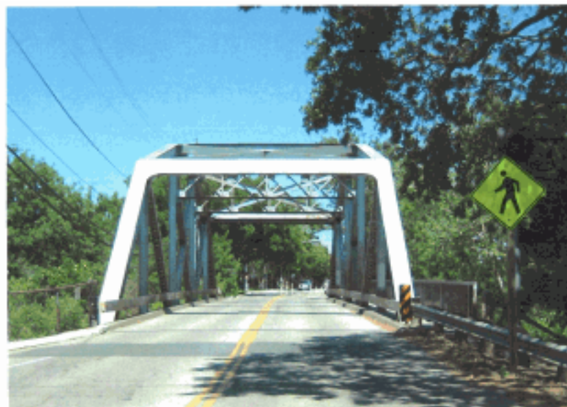
Bernal Avenue automobile bridge over Arroyo de la Laguna
