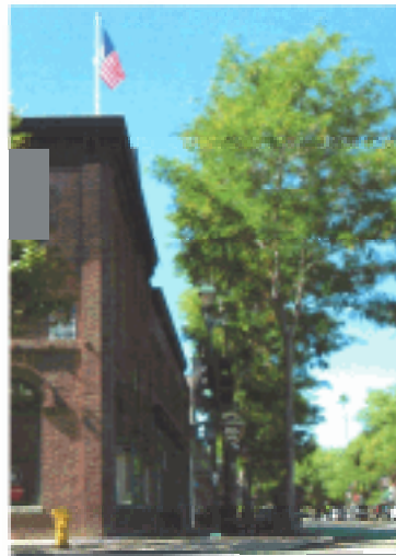
436-450 Main Street building
