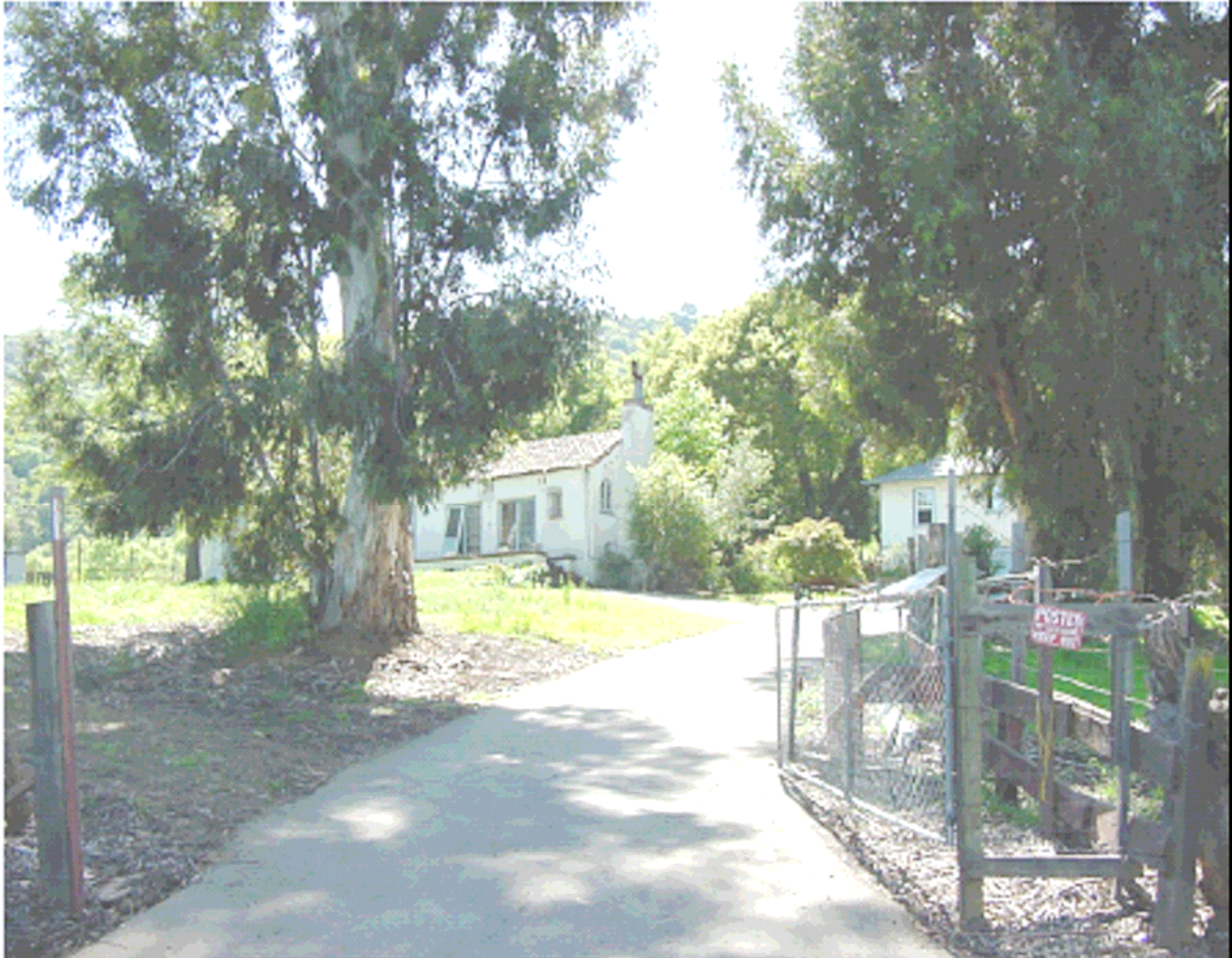
Figure 4: Caretaker’s home on Lot 7 and accessed from Old Foothill Road. The house will remain until vacated by the caretaker.
