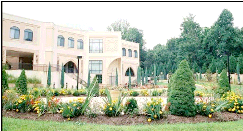
Landscaping at the MTO Virginia Facility
