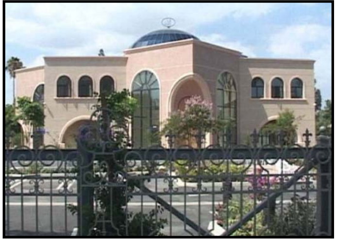
Front Elevation of Los Angeles Facility
