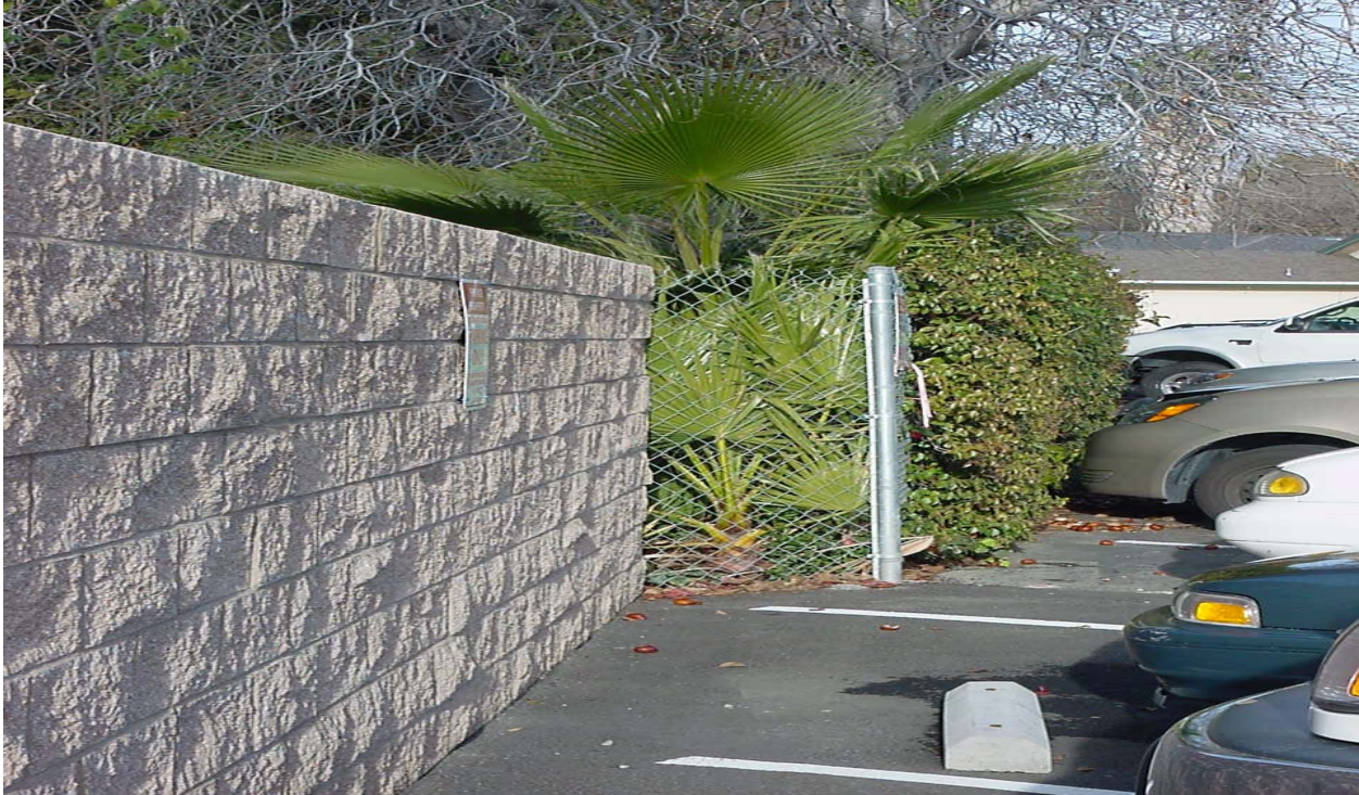
Figure 2, Transition from Masonry Wall to Vine Covered Chain Link Fence
