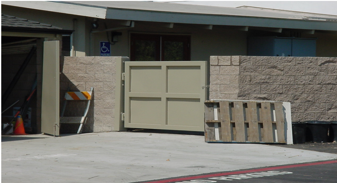
Figure 3, Gate from Haps to the Trash Enclosure
