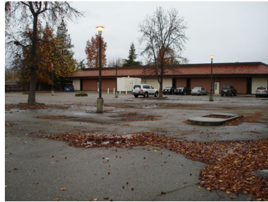
Rear Parking Lot
