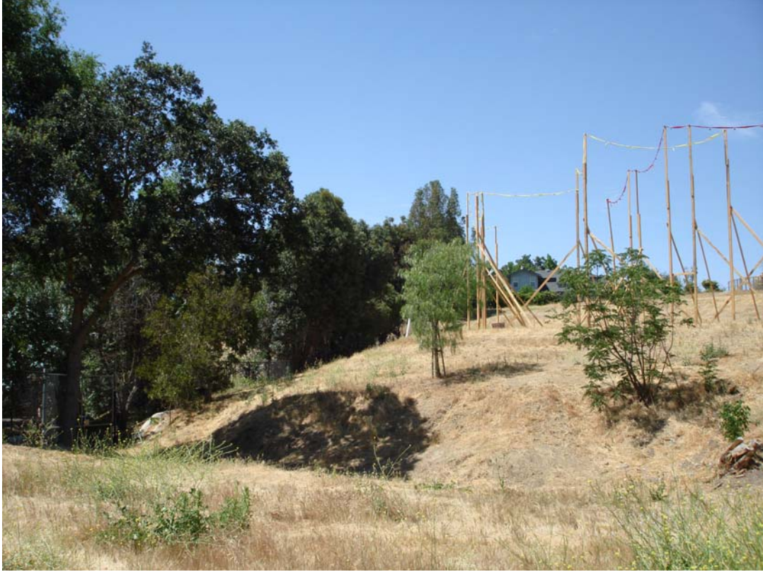
Figure 10: Story pole installation and Greene property.
