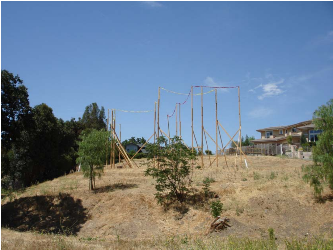
Figure 11: Story pole installation looking north from property line.
