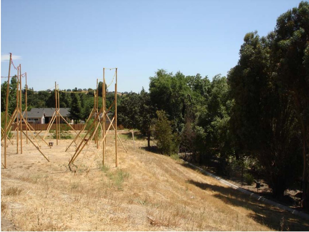
Figure 8: Story pole installation and Greene property.
