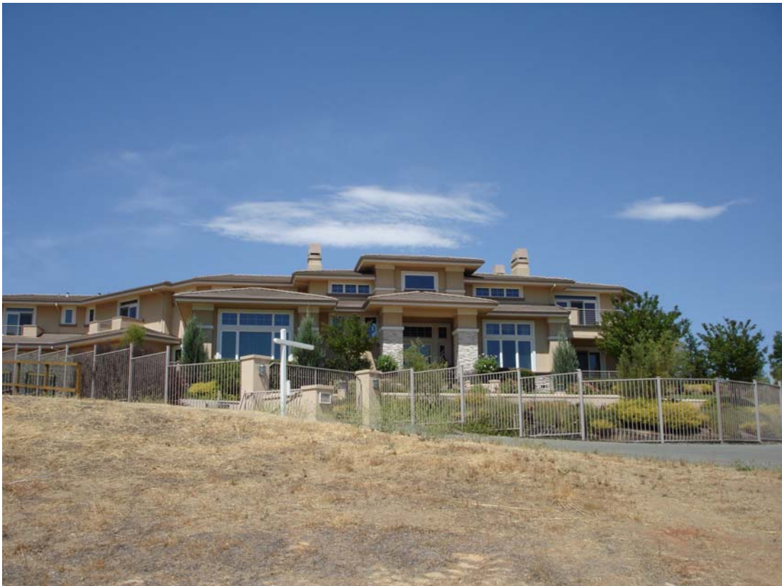
Figure 5: Bozorgzad home from the northeast side of the project site.
