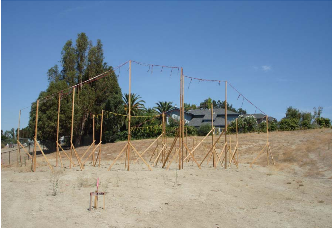
Figure 8: Story pole installation and the Ferrara property.
