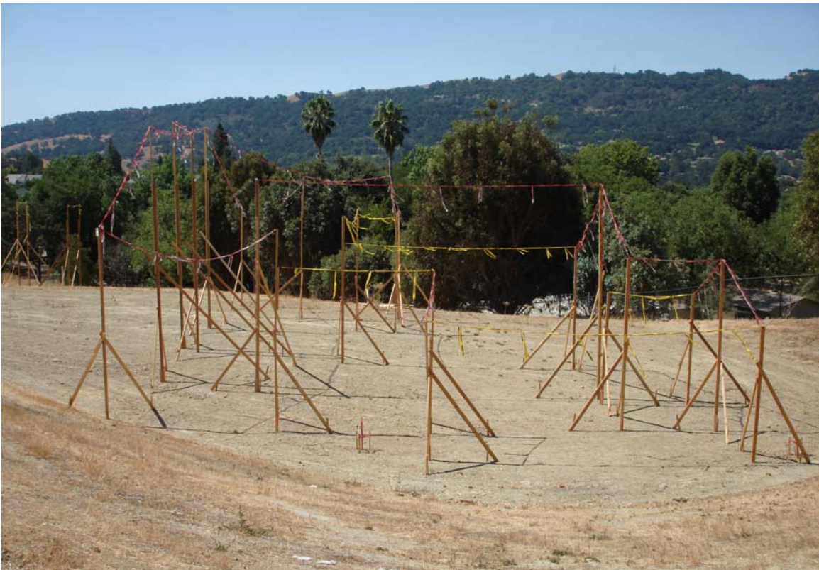
Figure 11: Looking through the east end of the home towards the Green property.
