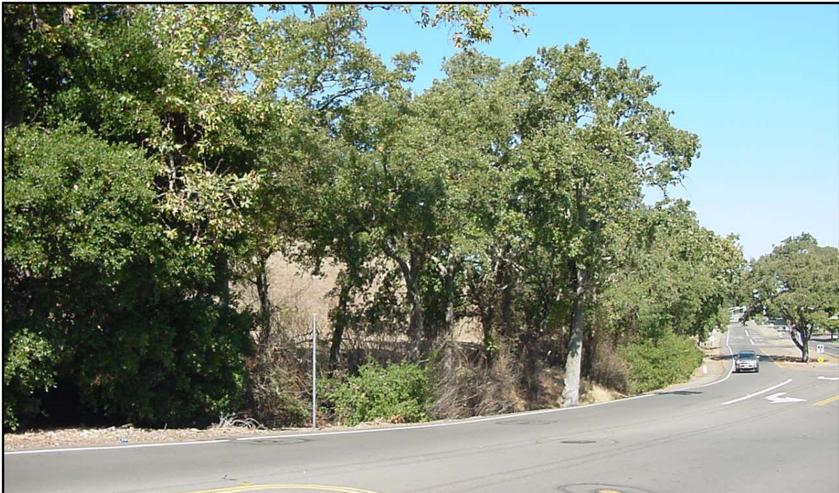
Figure 12: Section of Foothill Road where creek must be filled for bike lane.
