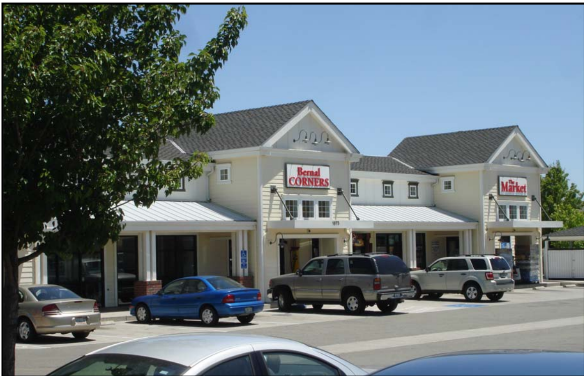
Figure 5: Bernal Corners Service Station from the Southside of Bernal Avenue.
