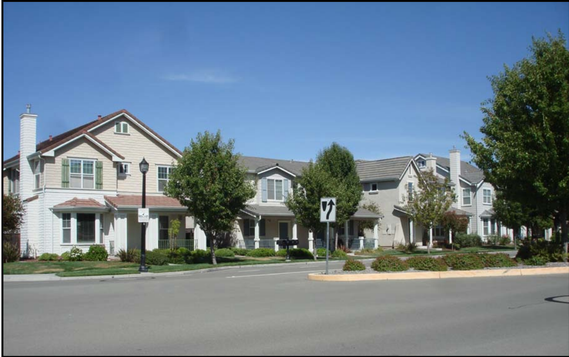
Figure 8: Walnut Hills Development from the West Side of Valley Avenue.
