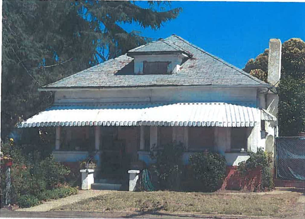
View of primary (south) façade, July 16, 2010 (Architectural Resources Group)
