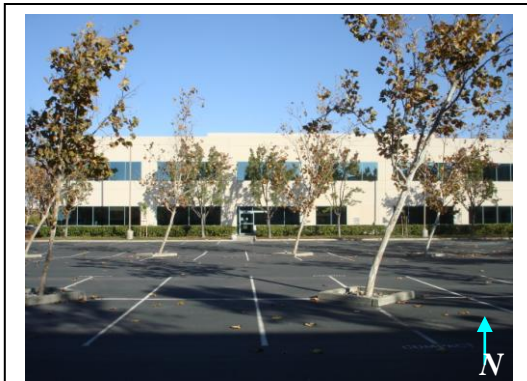
Photo 1.2: View of existing parking lot within the U-shape courtyard area.
