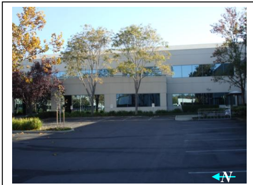
Photo 1.3: View of existing parking lot within the U-shape courtyard area.
