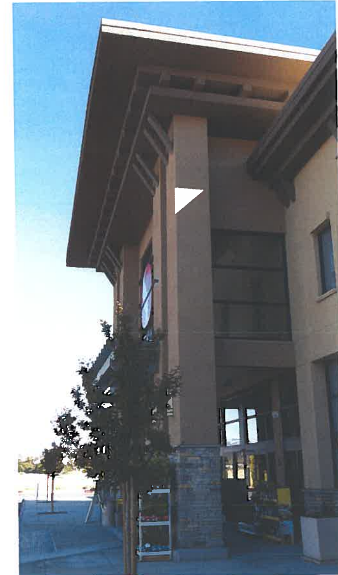
1 SAFEWAY STORE - MAIN ENTRY
