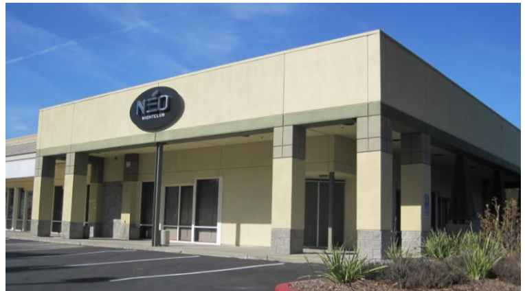
Photo 1.2 – South Elevation (secondary entry)
