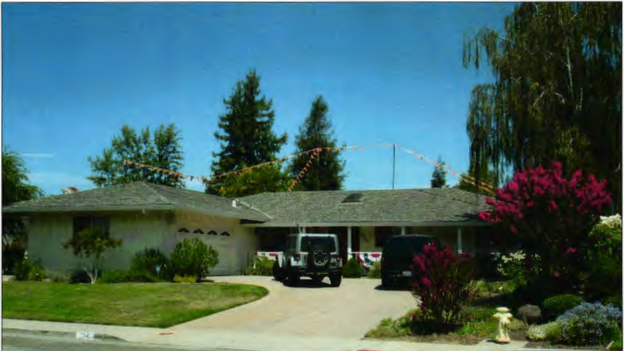
Figure 4 – Front View, 554 Hamilton Way
