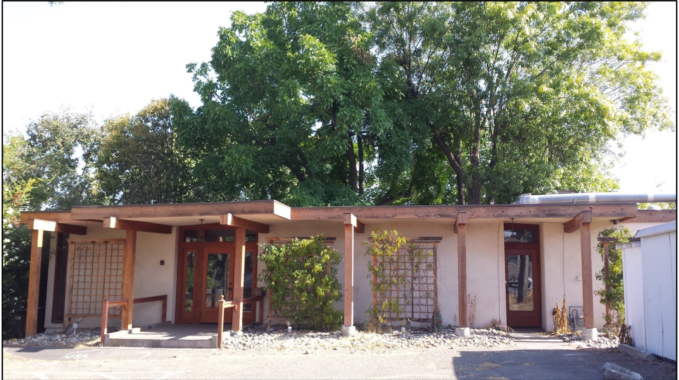
Figure 8: Existing building to be demolished
