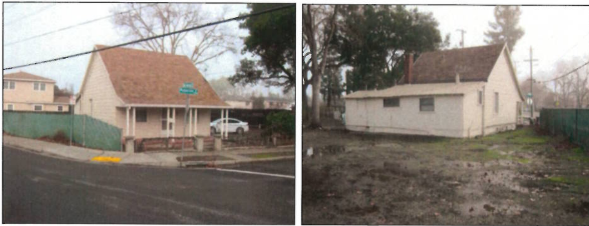
Figures 2 and 3. Left image shows the front and left side elevations of the residence. Right image shows the residence's rear elevation, with a poorly built and full-width rear addition.
