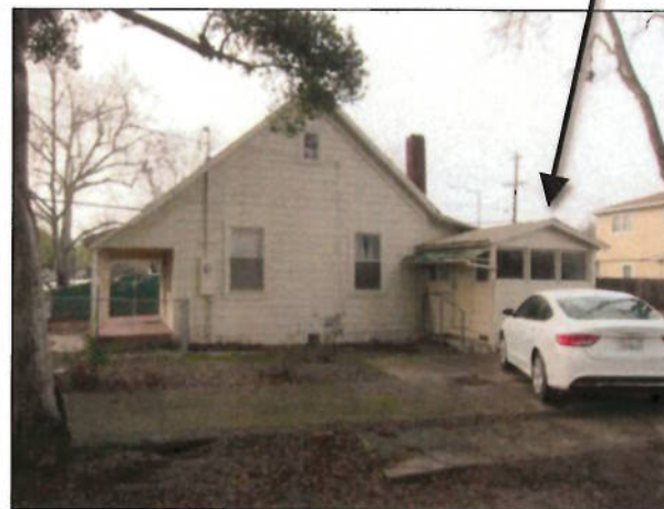
Figures 6 and 7. Left image shows the full width, front porch addition. Note the change in roof pitch that indicates where the porch's shed roof was connected to the main house roof (arrow). Right image shows the right side elevation, with an addition to the right side elevation shown with an arrow.
