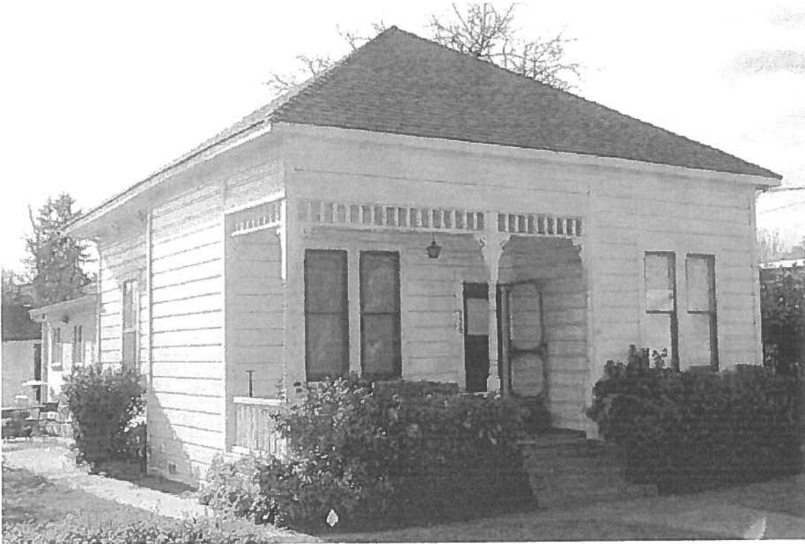
Fig.2 – 536 St. John St. - Left (east) side and Front (with non-historic porch addition at far left)
