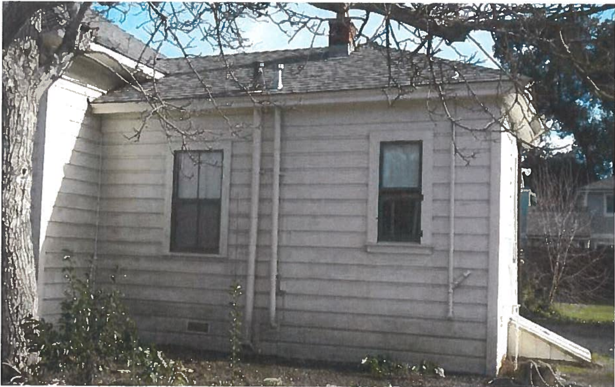
Fig.4 – 536 St. John St. - Rear structure at west side
