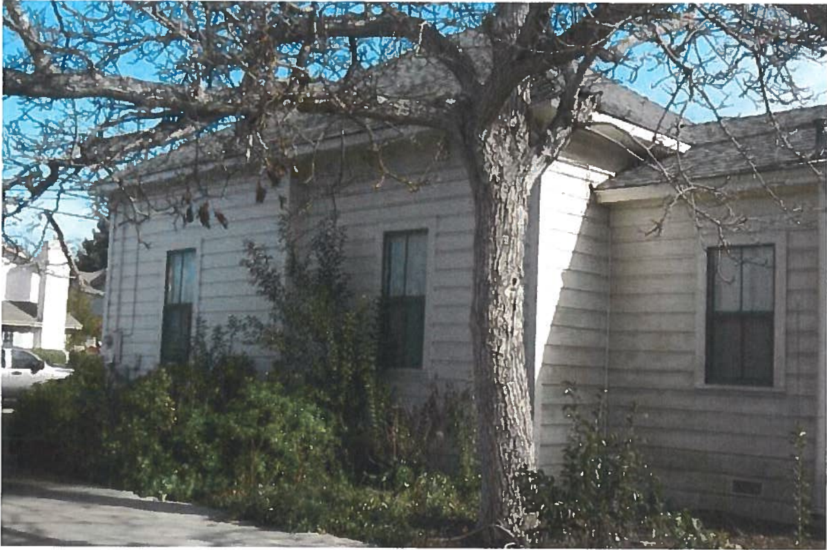
Fig.3 – 536 St. John St. - Front structure at west side
