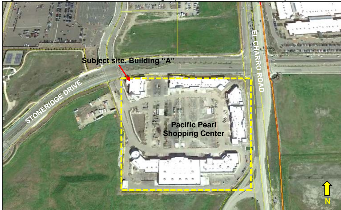
Figure 1: Google Earth Aerial Photograph ( Pacific Pearl is currently under construction )
