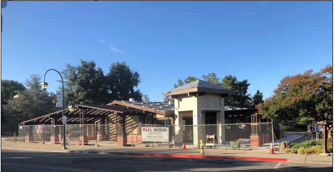
Figure 1: Current Building Under Construction
