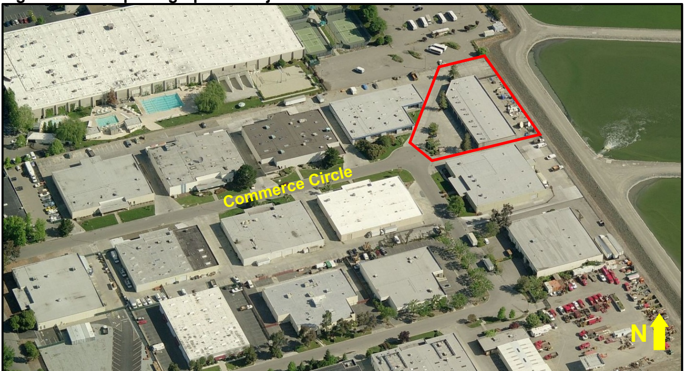
Figure 1: Aerial photograph of subject site
