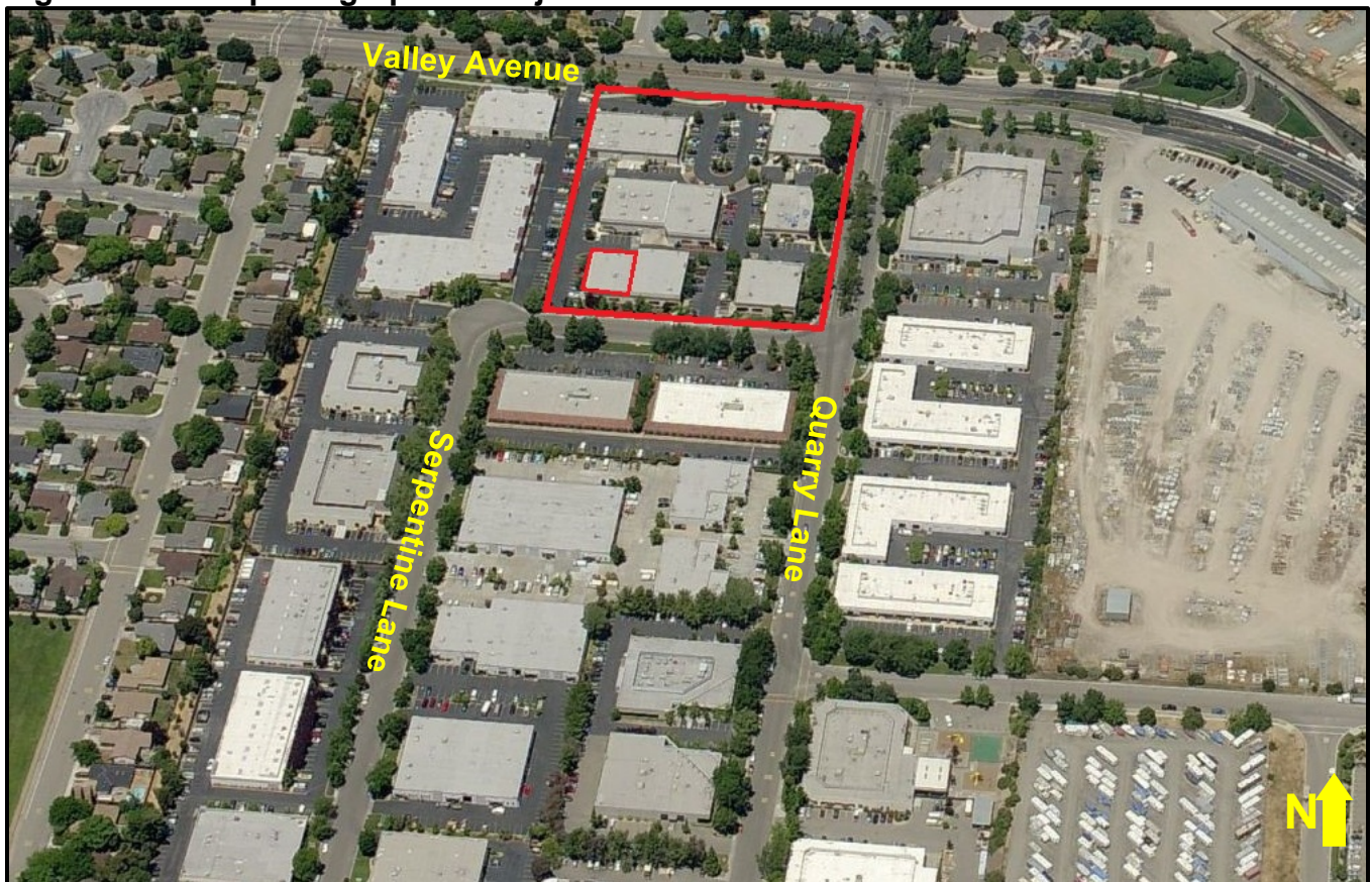
Figure 1: Aerial photograph of subject site
