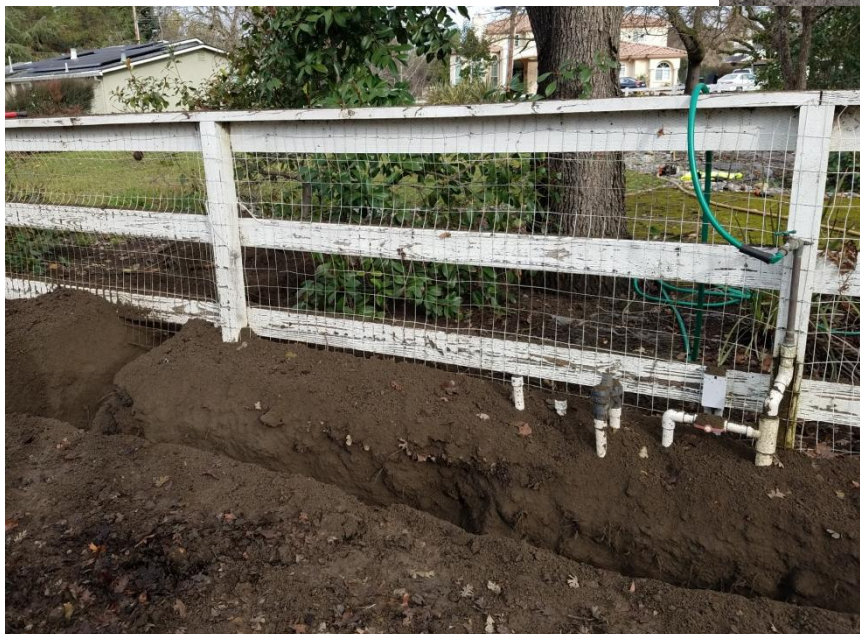
Figure 3. Exploratory trench by tree #23 was dug by hand with air spade assistance. Largest root measured 1.5" in diameter (above); all other roots were 1" or smaller. Roots were cleanly pruned before trench was backfilled.
