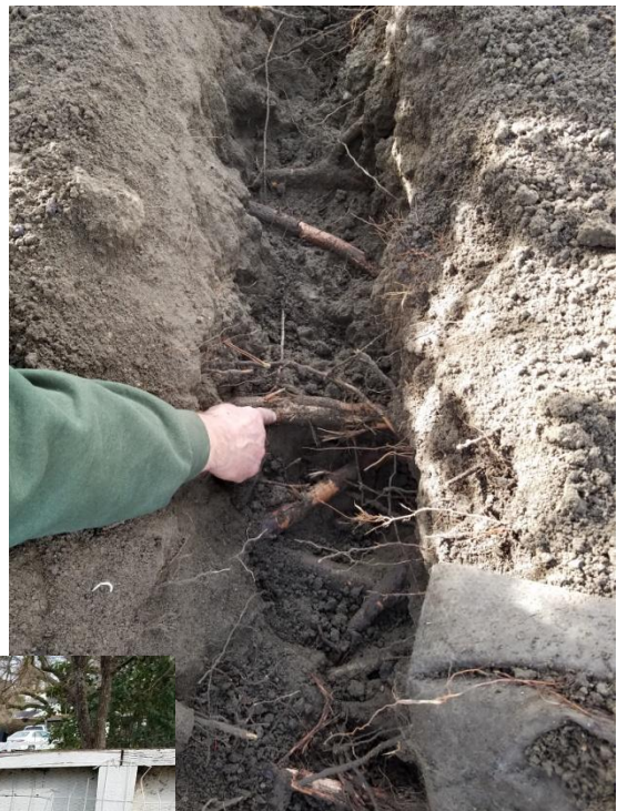
Figure 3. Exploratory trench by tree #23 was dug by hand with air spade assistance. Largest root measured 1.5" in diameter (above); all other roots were 1" or smaller. Roots were cleanly pruned before trench was backfilled.
