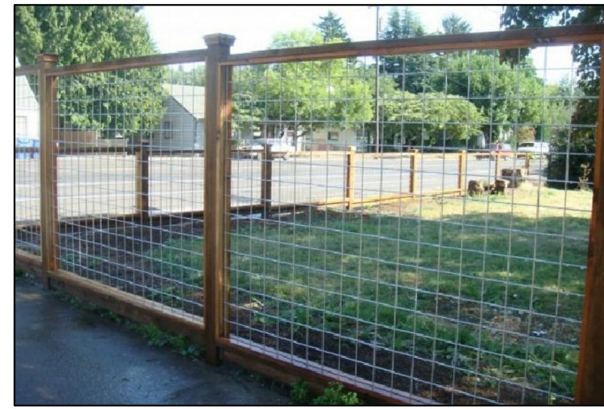
6' WELDED WIRE MESH FENCE
