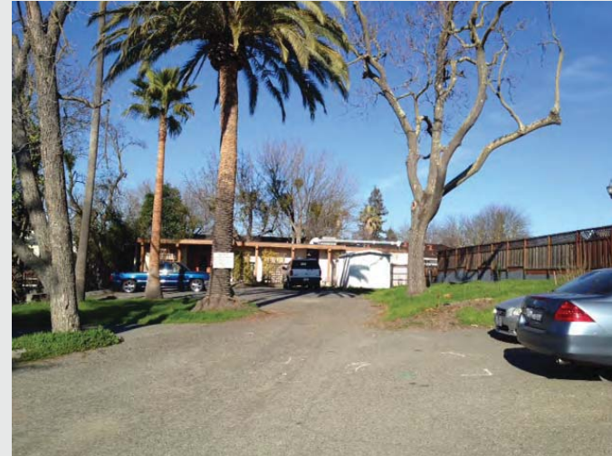
VIEW OF (E) STRUCTURE
