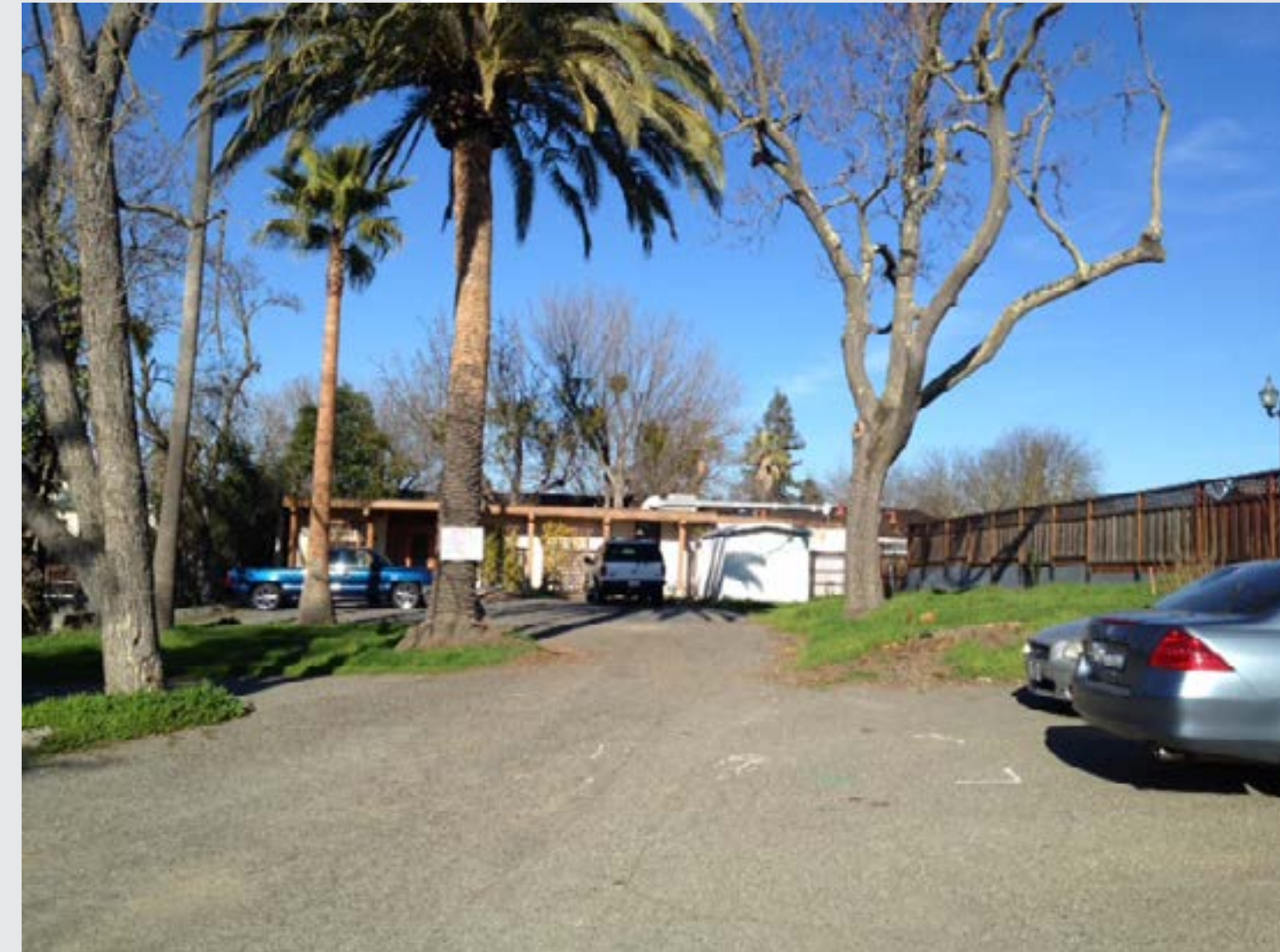
VIEW OF (E) STRUCTURE
