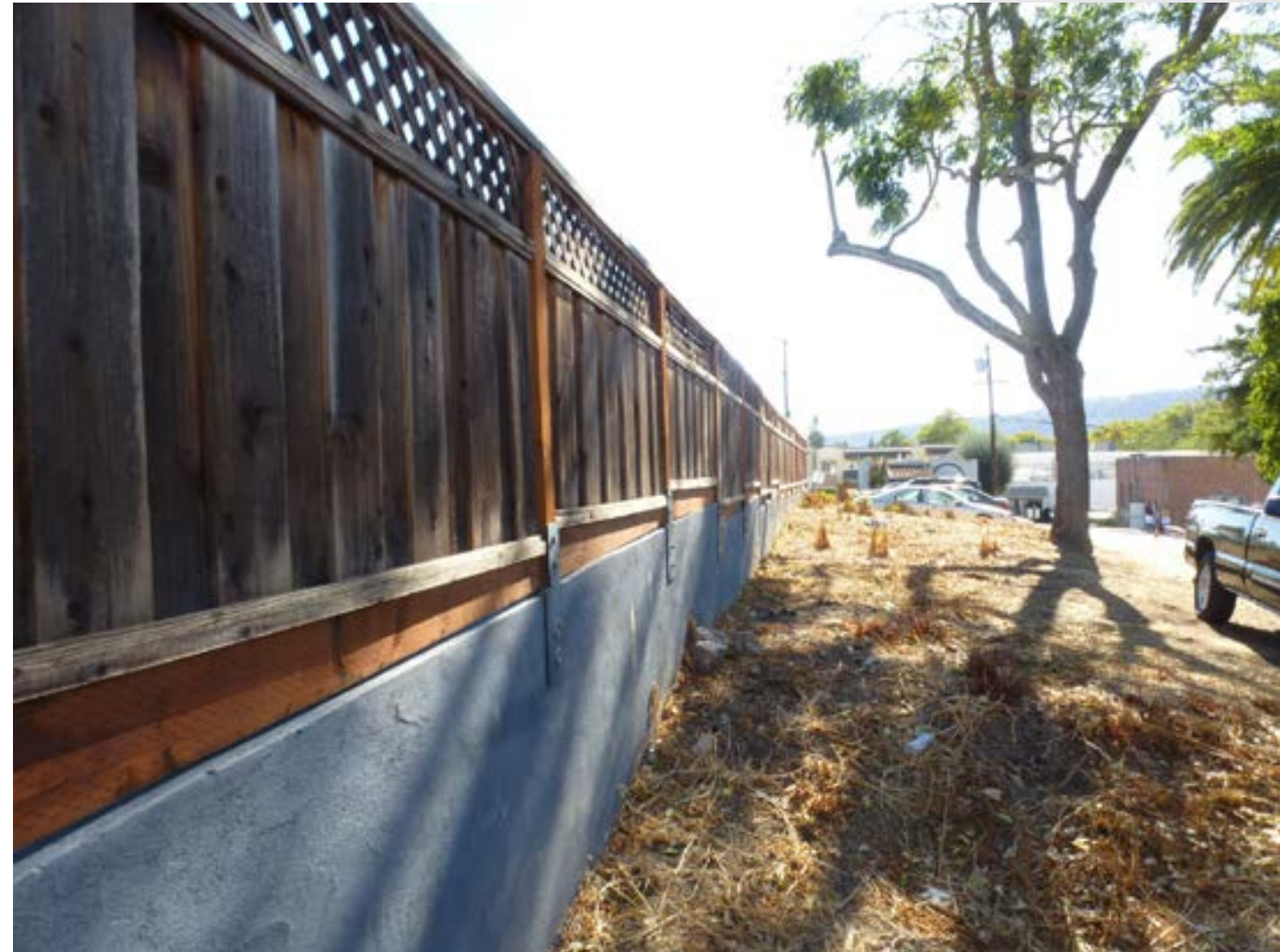
VIEW OF (E) FENCE @ EAST P.L.
