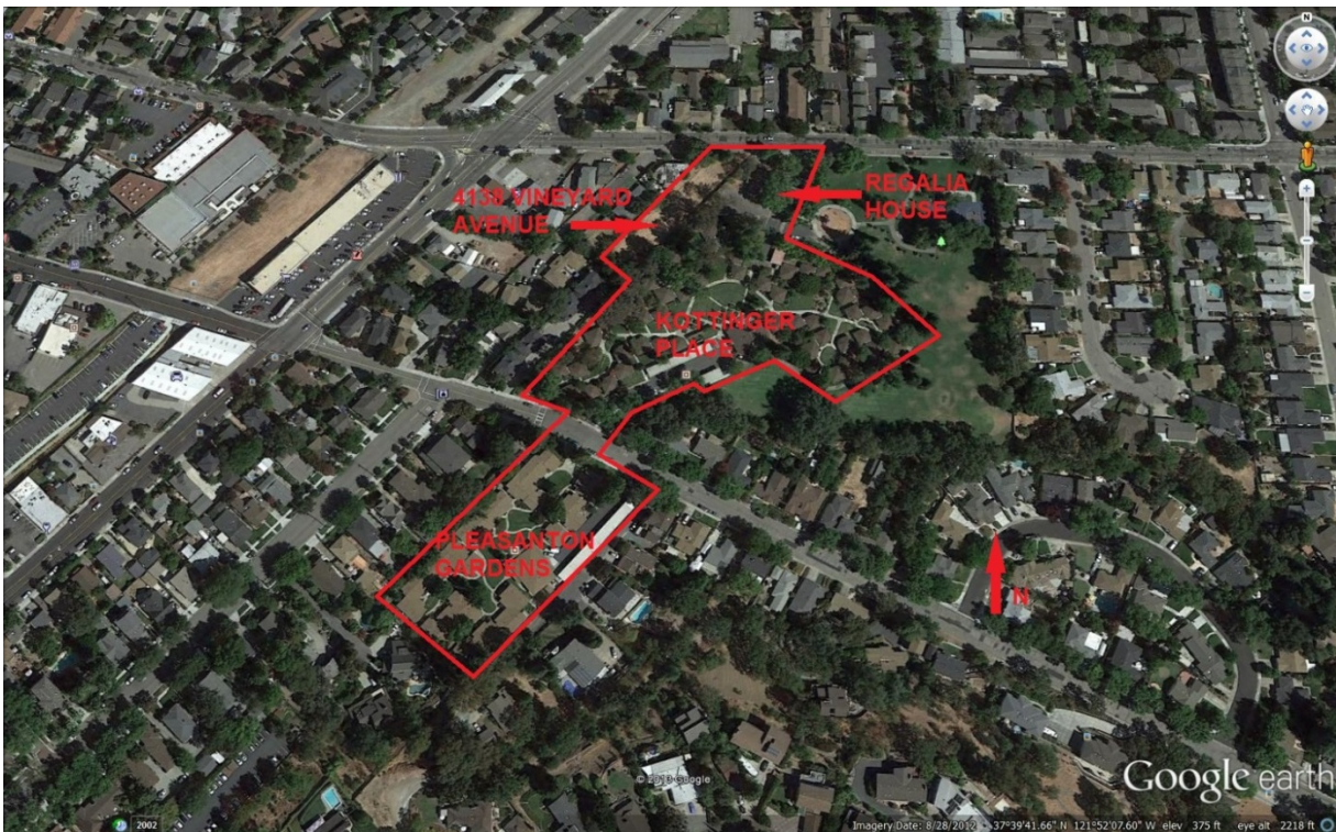
Aerial Site View
