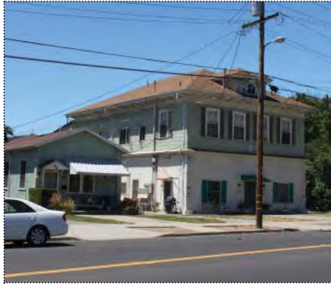
IDES Hall at 444 St. Mary Street (ARG, June 2012).
