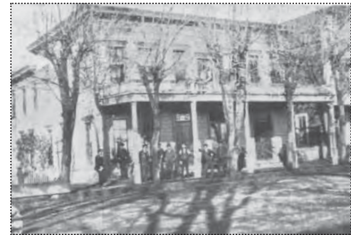
Built as the Germania Hotel in 1874, it was later known as the Pleasanton Hotel (demolished 1931) (from Pleasanton . Images of America, 50).
