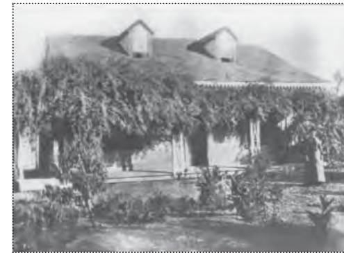
Adobe house built by John William Kottinger in 1852 (demolished 1930) (from Pleasanton . Images of America, 21).
