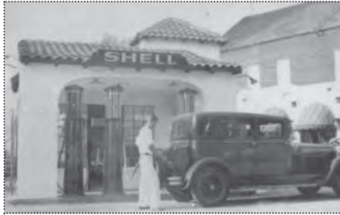
The J.J. Amaral Service Station and Garage were built in 1931 (from Pleasanton. Images of America , 123).
