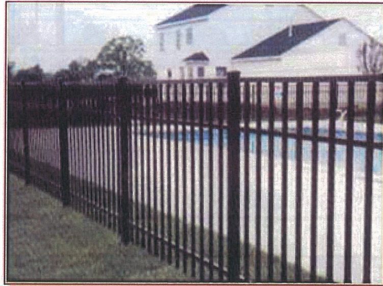
Typical Fence at CalTrans Right of Way
